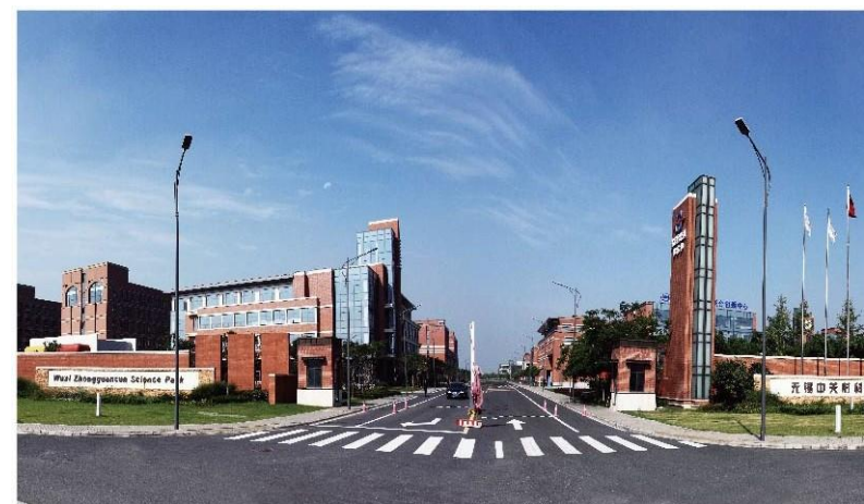
Wuxi Zhongguancun Science and Technology Innovation Park, a "high-end, low-carbon, environmentally friendly and ecological" high-tech industrial park
