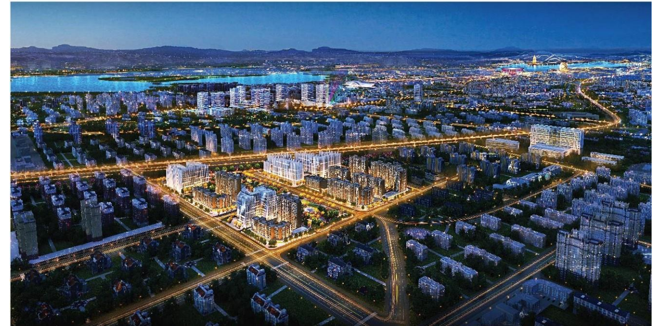
Beijing Huairou Science and Innovation Center Gateway to Huairou Science City, a platform for convergent industrial and business gatherings
